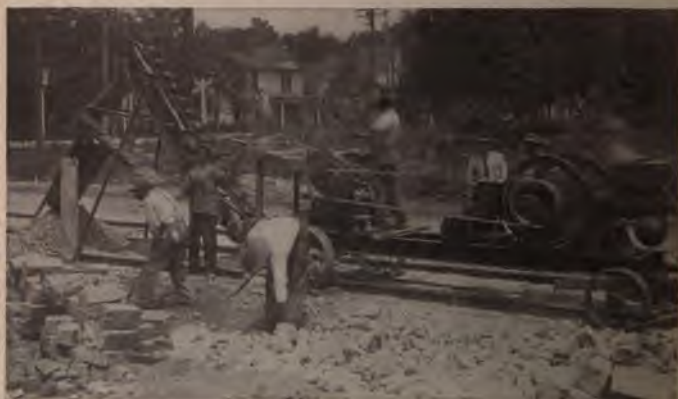
Crushing Old Stone Blocks for Concrete Base.
